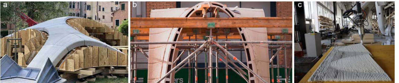
Figure 2: Existing approaches to robotic 3D concrete printing of vaulted and shell structures. (a,b) Discretized, prefabricated elements assembled on temporary internal scaffolding [44, 54]. (c) Directly printed self-supporting vaults relying on inherently stable geometries [52].
