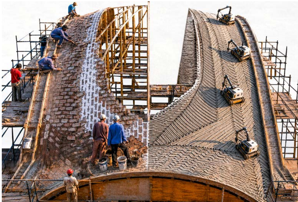
2 A speculative vision of the future of construction. Just as traditional brick vaults are assembled on site without scaffolding, guided only by lightweight timber centering, as shown on the left in Guastavino's method, concrete could one day be deposited in layers directly onto curved surfaces by multiple climbing robots, eliminating the need for formwork or scaffolding [right].
