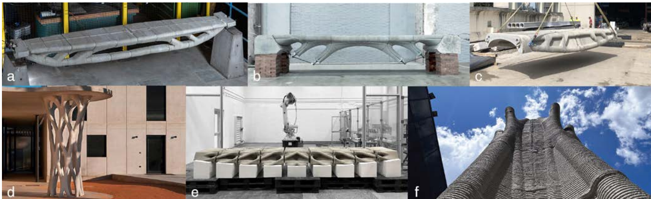
2 a: Topology optimized post-tensioned concrete girder (Vantghem et al. 2020); b: A cable-supported, unreinforced, and re-assemblable 3D printed concrete structure (Li et al. 2024); c: Topology optimized concrete footbridge (Ooms et al. 2022); d: Krypton, a column in Aix-en-Provence (Gaudillière-Jami et al. 2019); e: 3D printed, post-tensioned concrete canopy (Akbarzadeh et al. 2024); f: Topology optimized BranchWall. (Lin, Bayramvand, and Aghaei Meibodi 2025)
