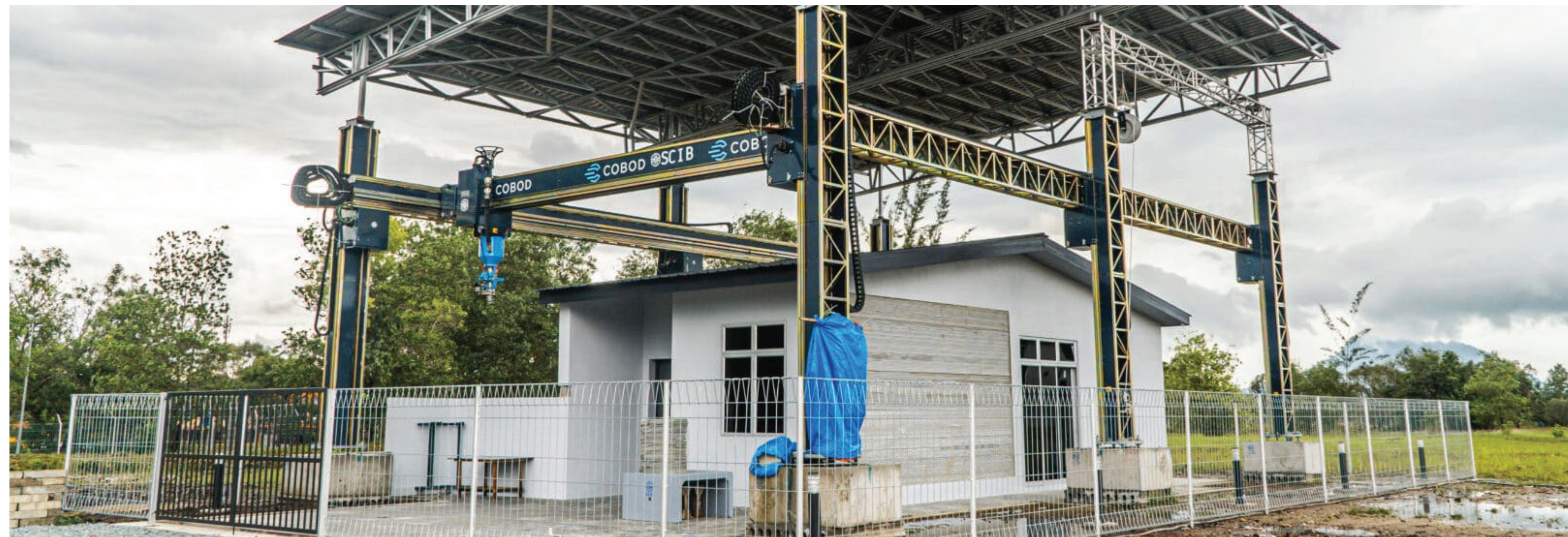
Figure 01: On-site gantry System for 3D Concrete Printing
