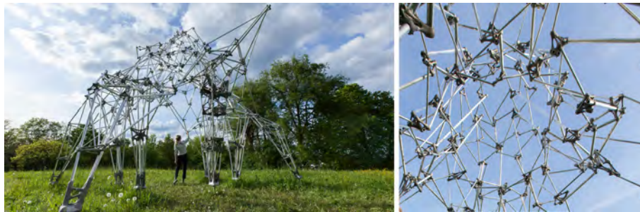
Figure 7. Liquid Metal Pavilion, space frame structure (left) and close up of nodes connecting aluminum tubes in variety of angle and position (right). Photographer: Demetris Shammas.
