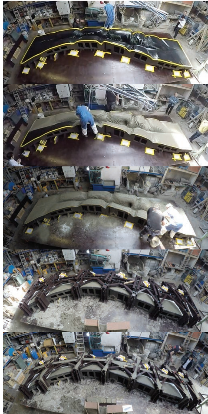
11. From top to bottom, (a) 3D printed formwork segment with release agent; (b) first concrete layer without fibers (sprayed); (c) 20mm thick concrete surface, spraying concrete on 3D-printed formwork segment; (d) Positioning pre-assembled timber formwork modules above the sprayed surface; (e) upstand beam cast inside the plywood formwork.
