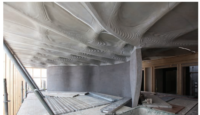
21 Interior view of the slab—ceiling. The scaffolding floor at mid room height facilitates assembly and improves safety
