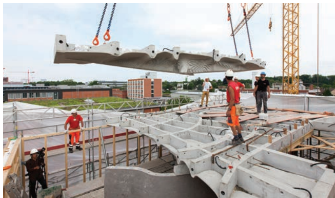
20 On-site assembly of concrete segments.
