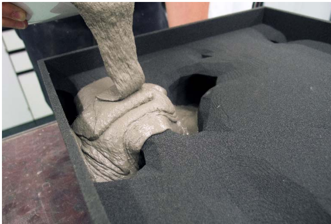
Figure 12. Casting UHPFRC inside the 3D-printed formwork.
