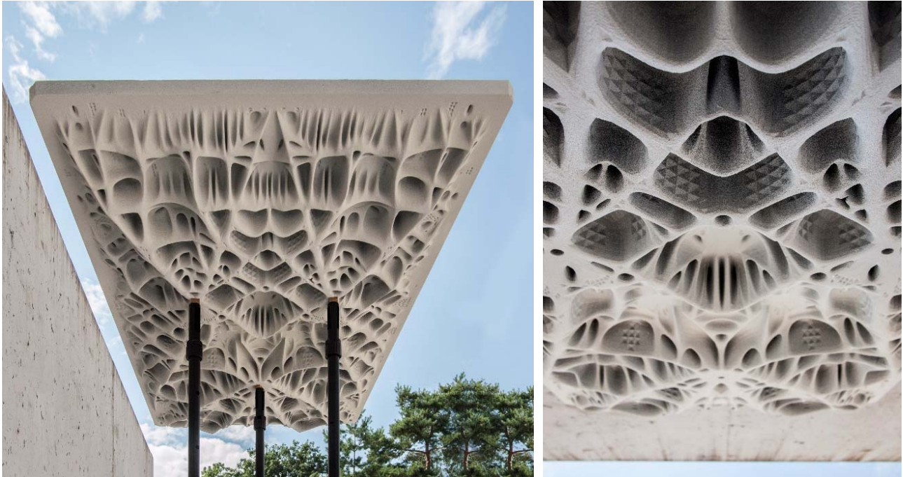
Figure 4, left. Prototype “A”; topology optimization of a slab with three supports.
