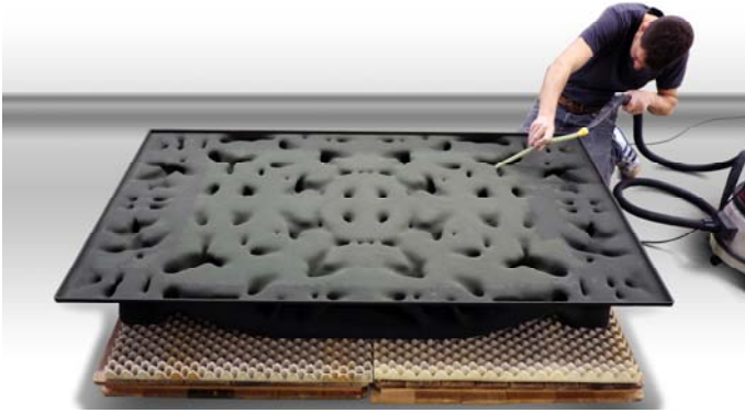
Figure 11. Post-processing of the 3D-printed formwork.
